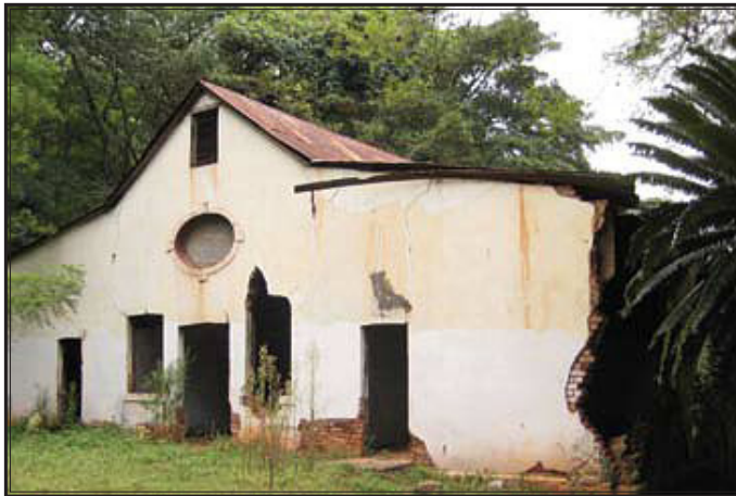
Fig 1: The remaining building of Lemana Training College in 2013.
